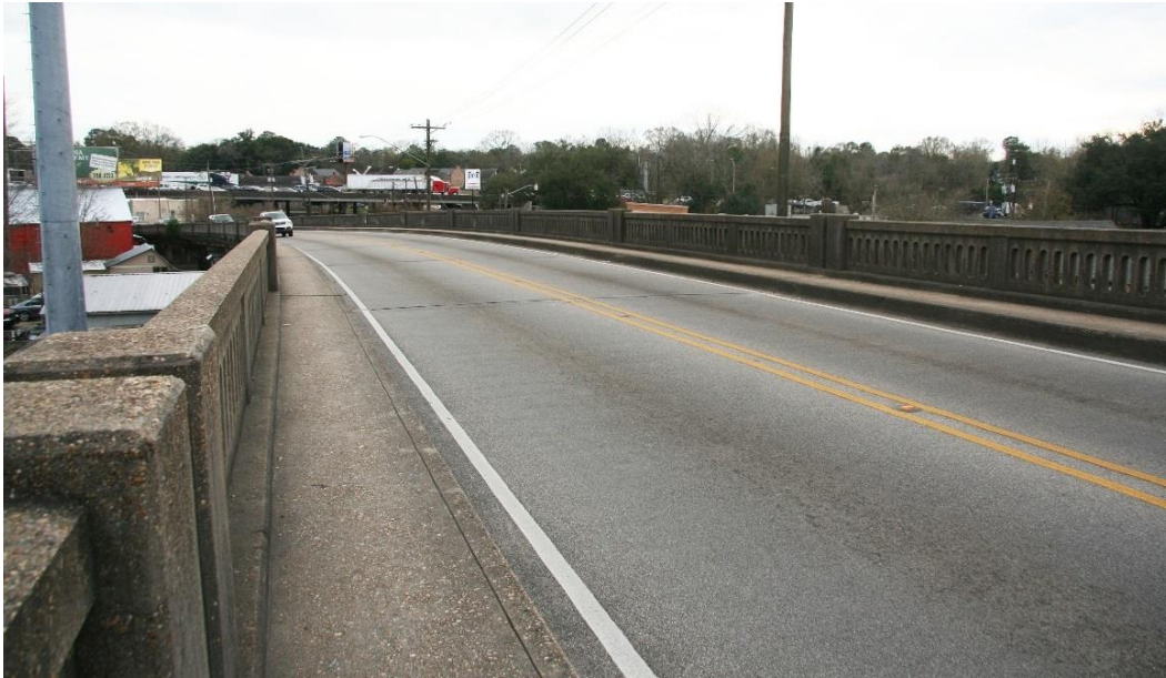
Condition Photo 9: General condition of bridge deck, sidewalks, and railings.
