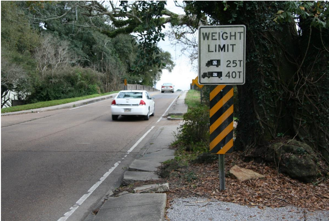
Condition Photo 13: North end of bridge approach roadway, including sidewalk.
