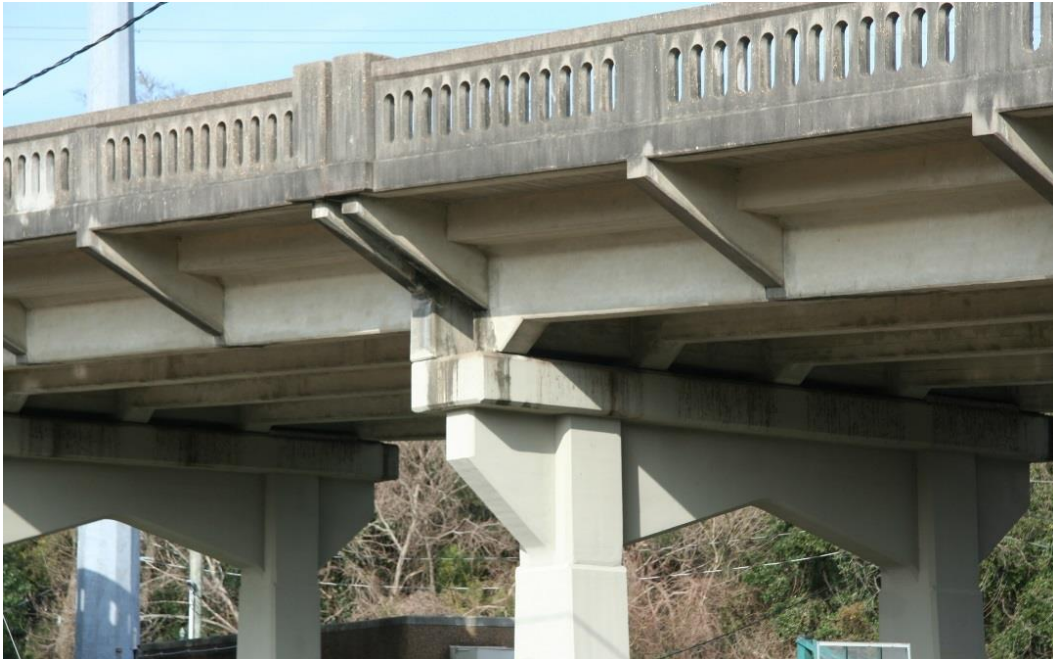
Condition Photo 3: Typical superstructure and pier.
