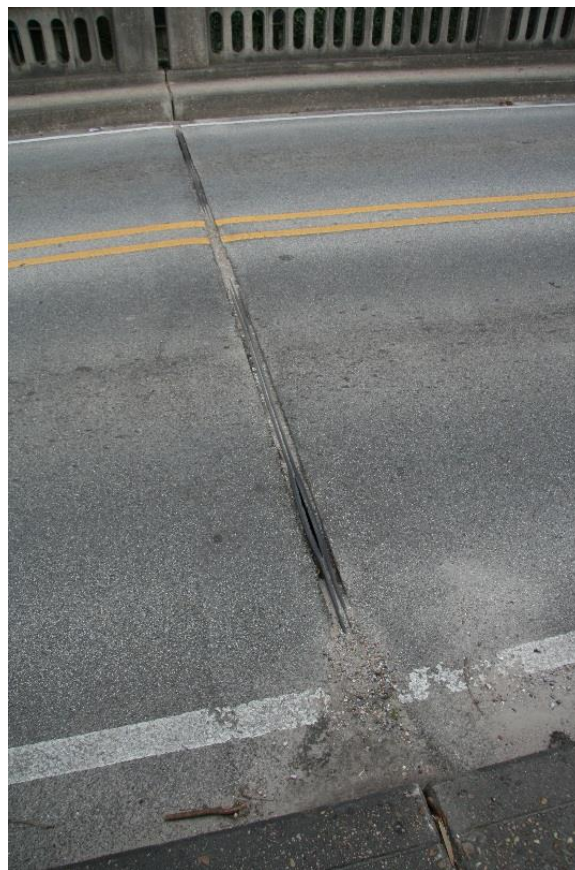
Condition Photo 10: Typical roadway expansion joint in approach spans.
