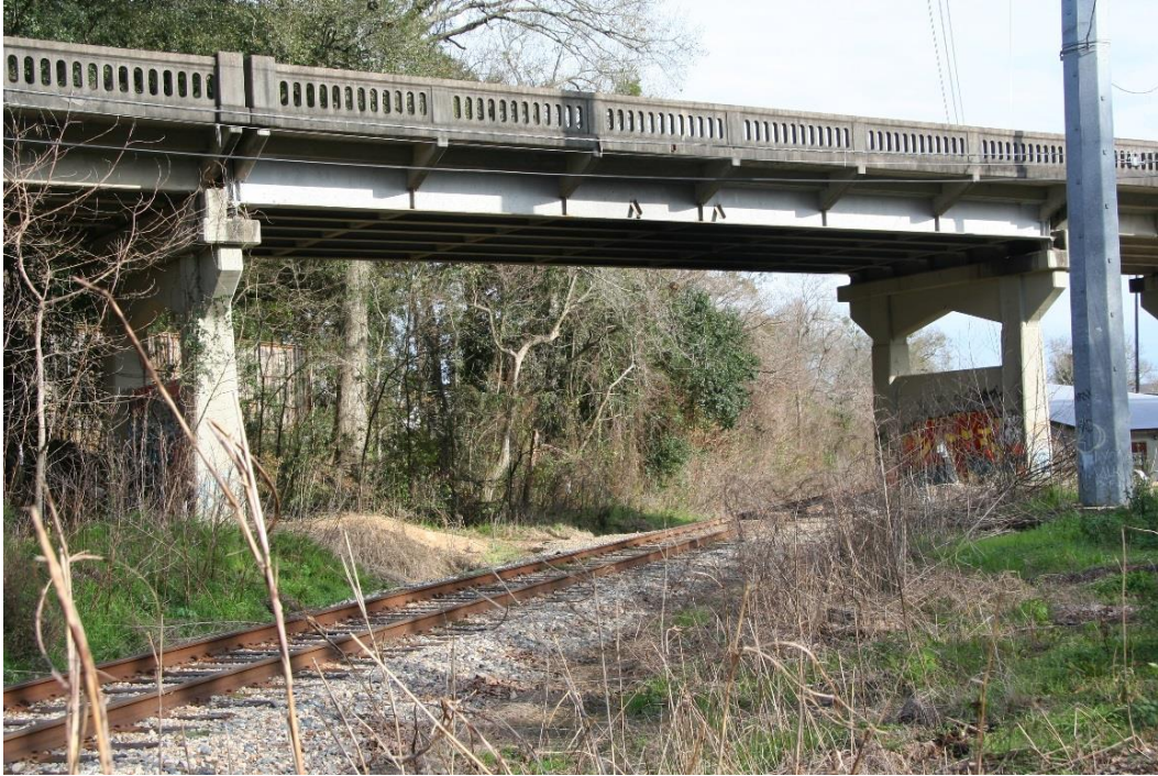
Condition Photo 5: Steel I-Beam span over railroad.
