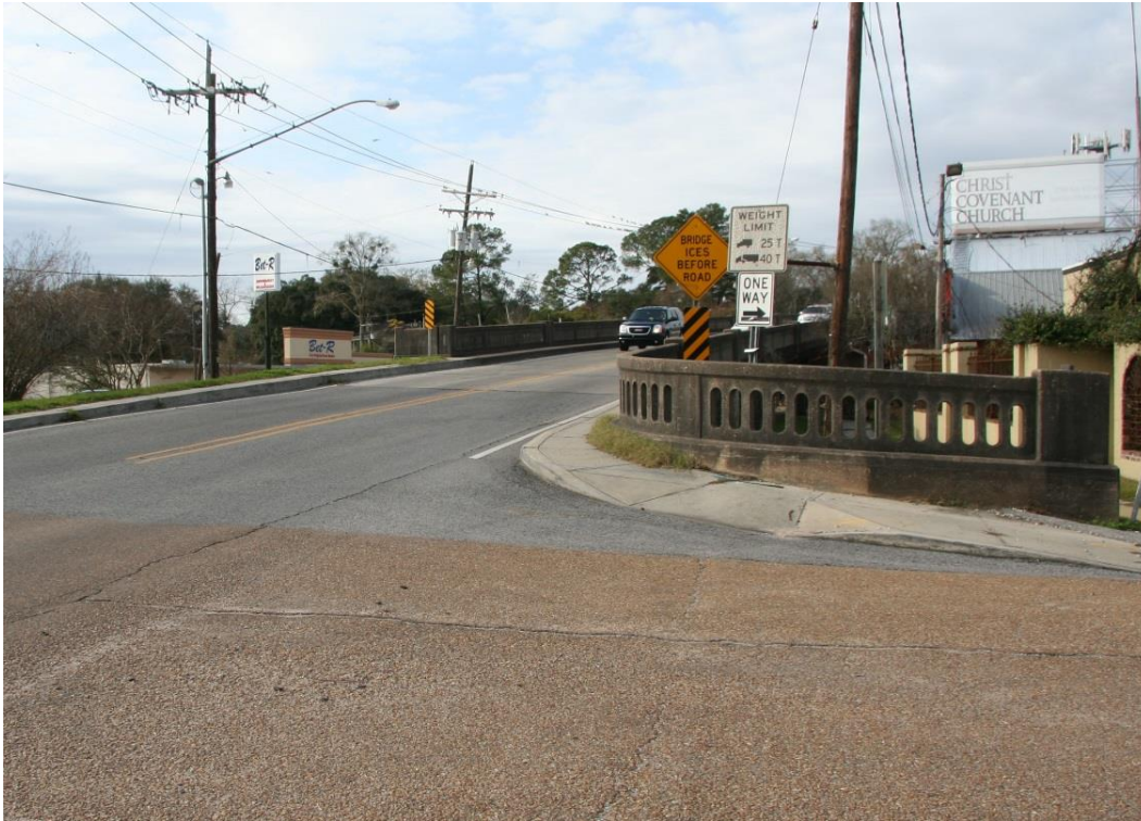
Condition Photo 1: South end of bridge approach roadway and bridge railing.
