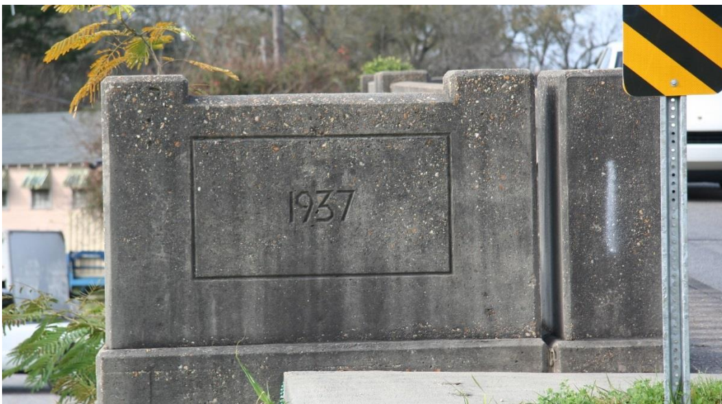
Character-defining Feature Photo 4: Aesthetic treatment of geometric endposts contributes to the overall design treatment of the overpass.
